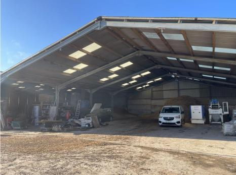
buildings. The buildings each measure approximately 80' x 60' (4,800 sq ft) and are of steel portal frame construction with concrete floors and walls with pitched corrugated fibre cement roof coverings. Additional planning permission exists for a 20m x 40m all-weather equestrian menage and a further 24m x 10m agricultural shed on the yard. As such, the property may suit equestrian buyers as in addition to the all-weather menage permission there is a further 24 acres of grazing land.
